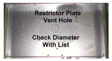
On any service calls for pressure switch not making or nuisance tripping, limit and/or rollout nuisance tripping on 80% Tubular Furnaces within Serial Number Range W0L6 (Oct 2006) to W0C7 (Mar 2007) with a nuisance limit or roll out tripping problem. York will provide one-hour labor allowance per unit for inspection to verify the hole size and another hour to replace wrong restrictor plate with correct one if needed.
